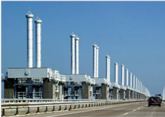
Figure 5.3 New road on the Oosterscheldekering
