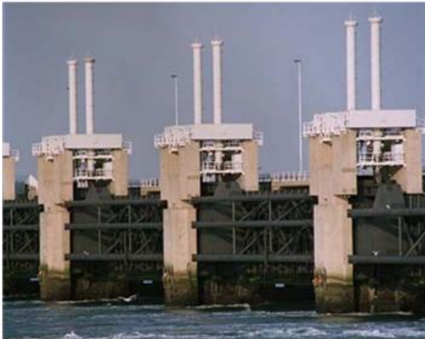
Figure 5.2 Movable barriers in the Oosterscheldekering
