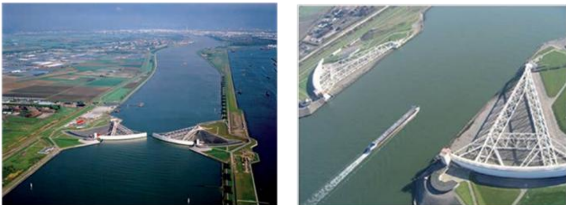
Figure 5.6 Maeslantkering: open (left) and closed (right)
